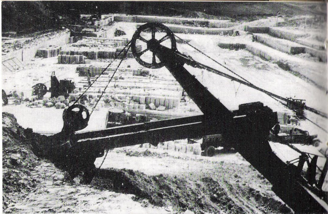
The excavator in the foreground is stripping the earth from the layer of building stone—a type of limestone—beneath. Machines are slicing the stone into blocks, and lorries take these direct to the building site.
