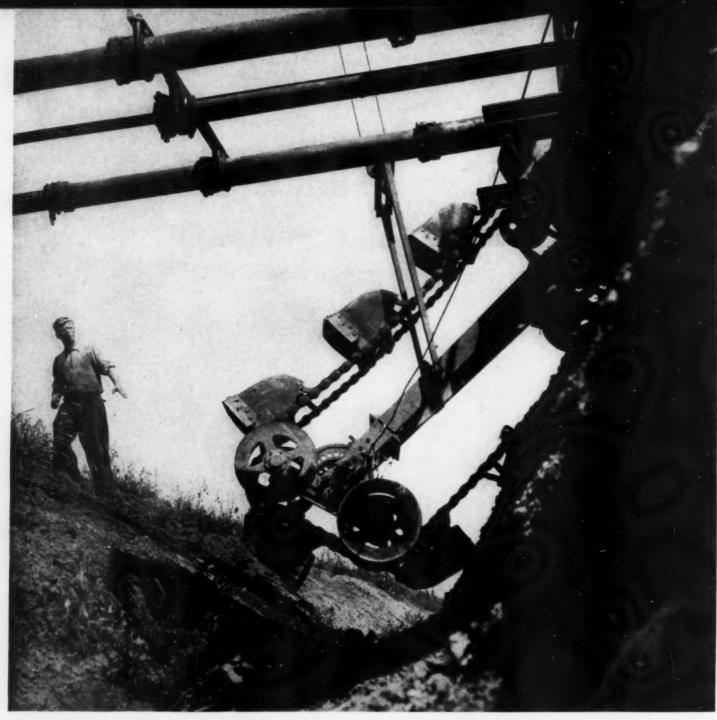
MULTI-BUCKET EXCAVATOR MAKES SHORT WORK OF TOUGH DIGGING AND SOON HAS A DRAINAGE CANAL COMPLETED TO RECLAIM ACRES OF RICH FARMLAND FOR CROPS.
