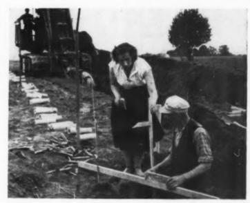
DRAINAGE TILE IS BEING LAID UNDERGROUND IN SWAMPY LITHUANIAN FIELDS.
