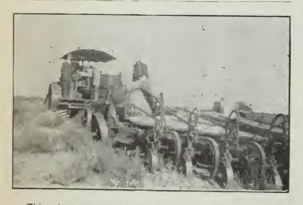
This giant tractor, with two men in charge, clears ten acres of land a day. It mows down monster "joshua" trees, greasewood and sage in an astonishing manner. These tractors are also used for digging irrigation ditches on the Llano property. It digs a ditch three feet deep and two feet wide as it sweeps steadily and irresistibly along the lines marked out by the surveyors. All of the plowing will be done by these machines.
