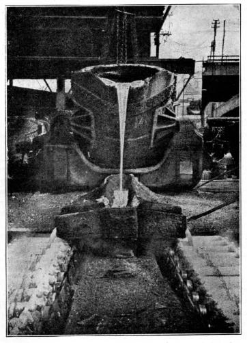
FRONT VIEW OF LADLE EMPTYING MOLTEN METAL INTO MOLDS,
